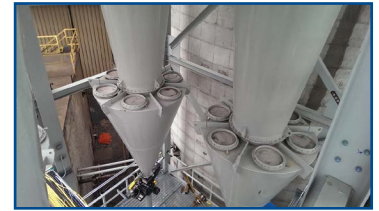
Fisher-Klosterman Emtrol Ultra high efficiency cyclones with explosion vents
