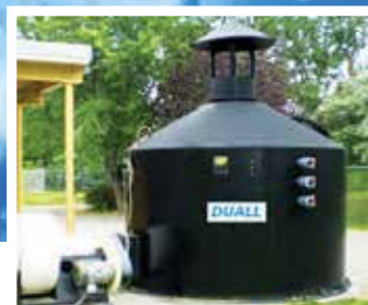
Carbon Canister with Integral Fan
