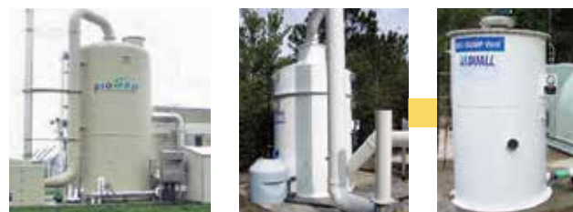
Biotrickling Filter Removing Odors
